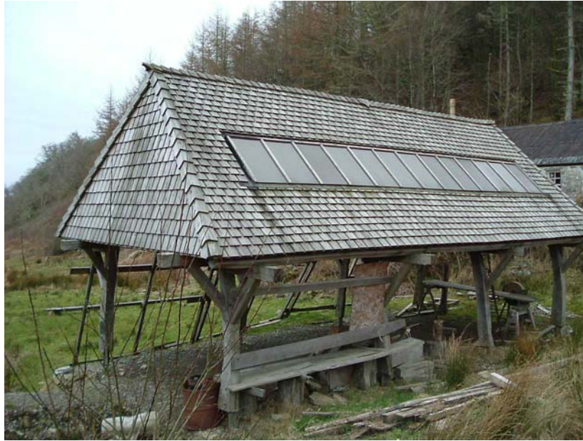
Fig 2. Pre-dating the log loo is an adjacent cruck-frame oak shelter for holding workshops
