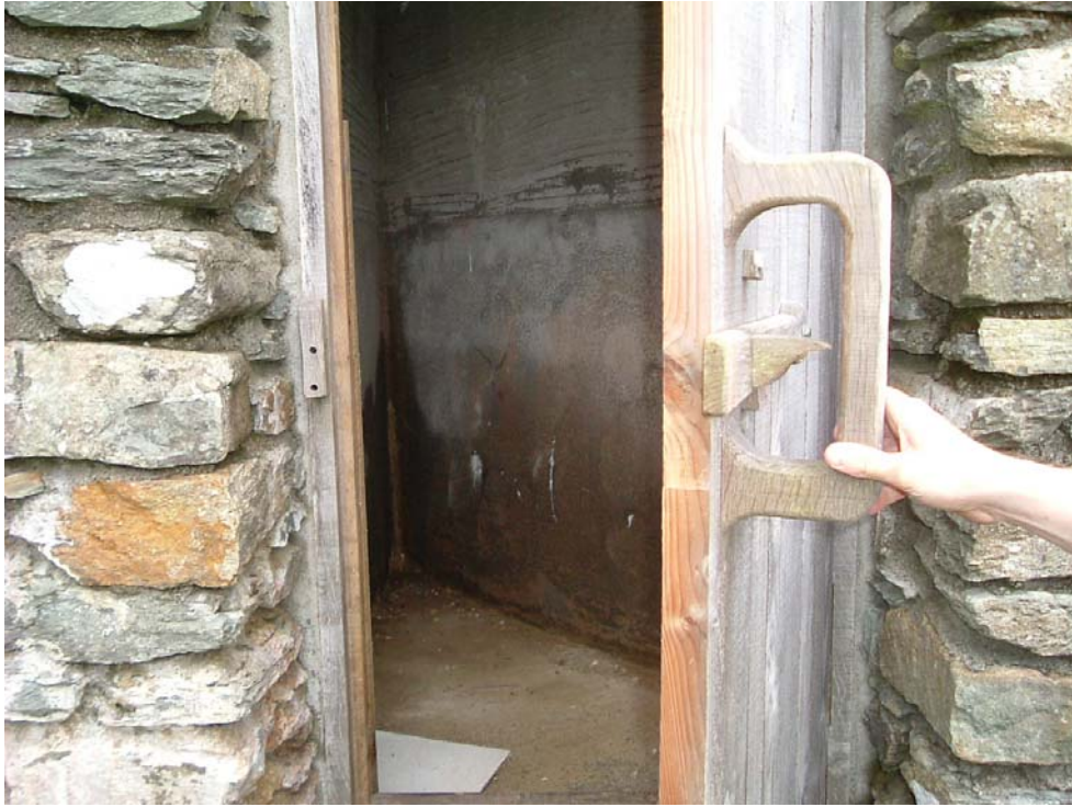
Fig 5. One of the stone-built, concrete-lined understorey compartments
