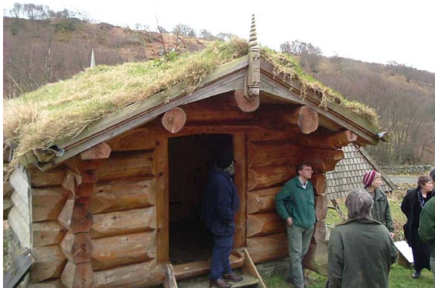
Fig 3. Sunart Oakwoods Initiative visitors to Barnluasgan admire the construction
