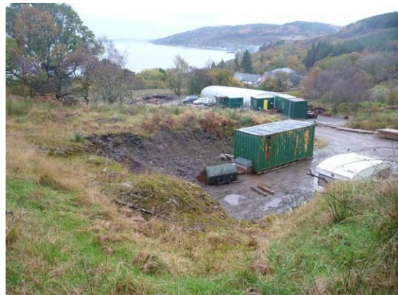
View from above the main working area
