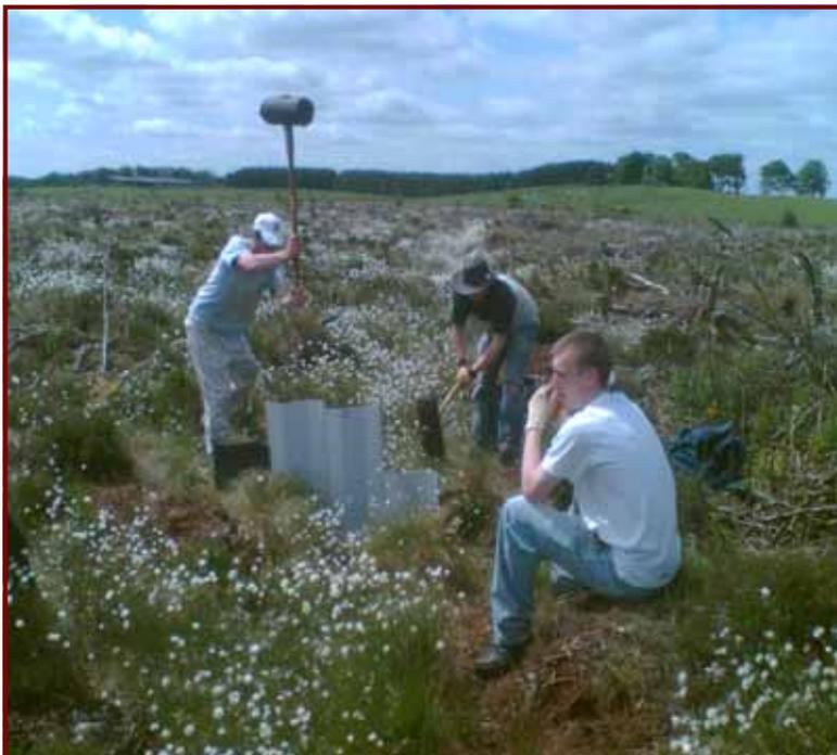
Each dam was constructed of lengths of interlocking plastic piling, up to 3 metres in length which were hammered into the ground to create a watertight dam. The team used clearing saws to remove regenerating tree species, particularly lodgepole pine, which were encroaching from surrounding woodland.
